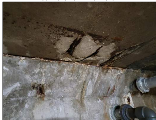
32. EXPOSED REBAR IN TUNNEL AND PRECIPITATE.
