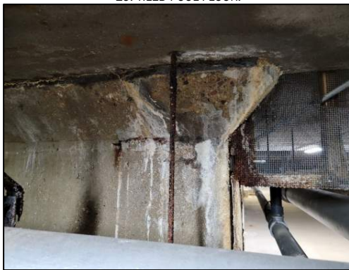
31. CONCRETE DETERIORATION.
