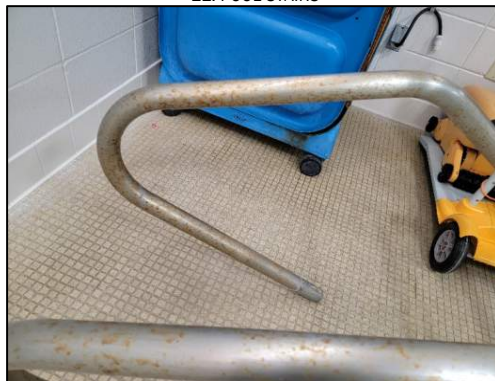
13. POOL LADDER CORROSION.
