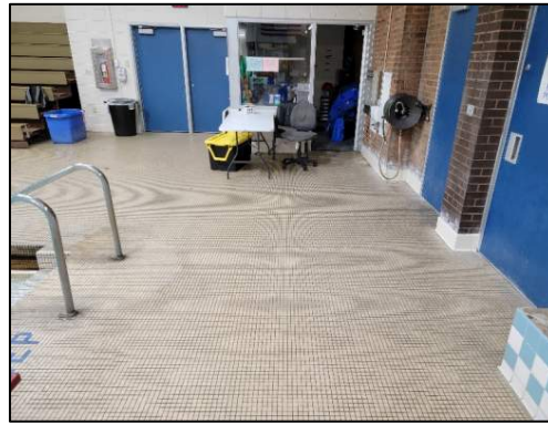
4. POOL DECK BY ENTRANCE TO SCHOOL
